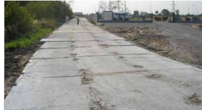
Kolomna / Port Construction 1.2 Km Road Building
